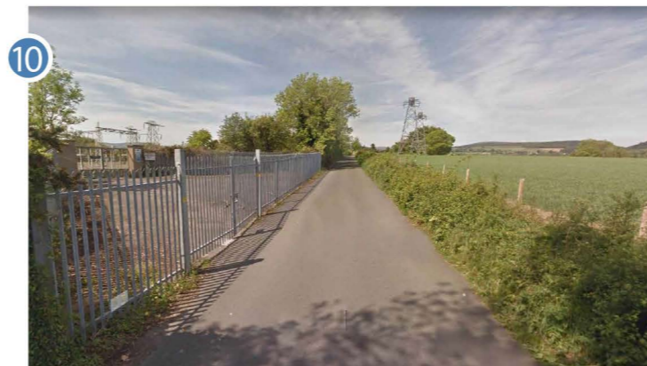
Berryfield Lane at ESB substation looking west
